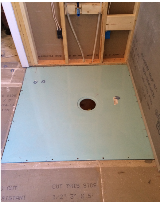
Classic shower base installed on joists.
